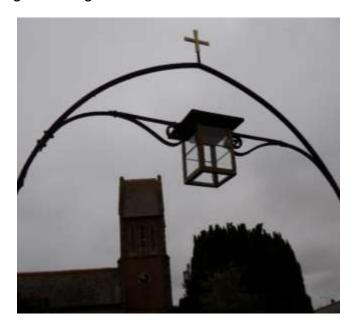
There was originally an oil lamp which fitted into the square holder in the arch above the gate, but this disappeared many years ago. The wrought iron arch probably dates from 1867 when the church building was altered and the saddleback top was added to the tower. The new lamp fits into the same holder and is of a simple design to complement the original arch and the church building.
